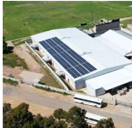
The Caledon manufacturing facility installed a 100 kWp photovoltaic system in 2016.
