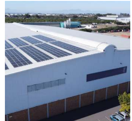
The Tygerberg distribution centre installed a 178 kWp photovoltaic system in 2024.
